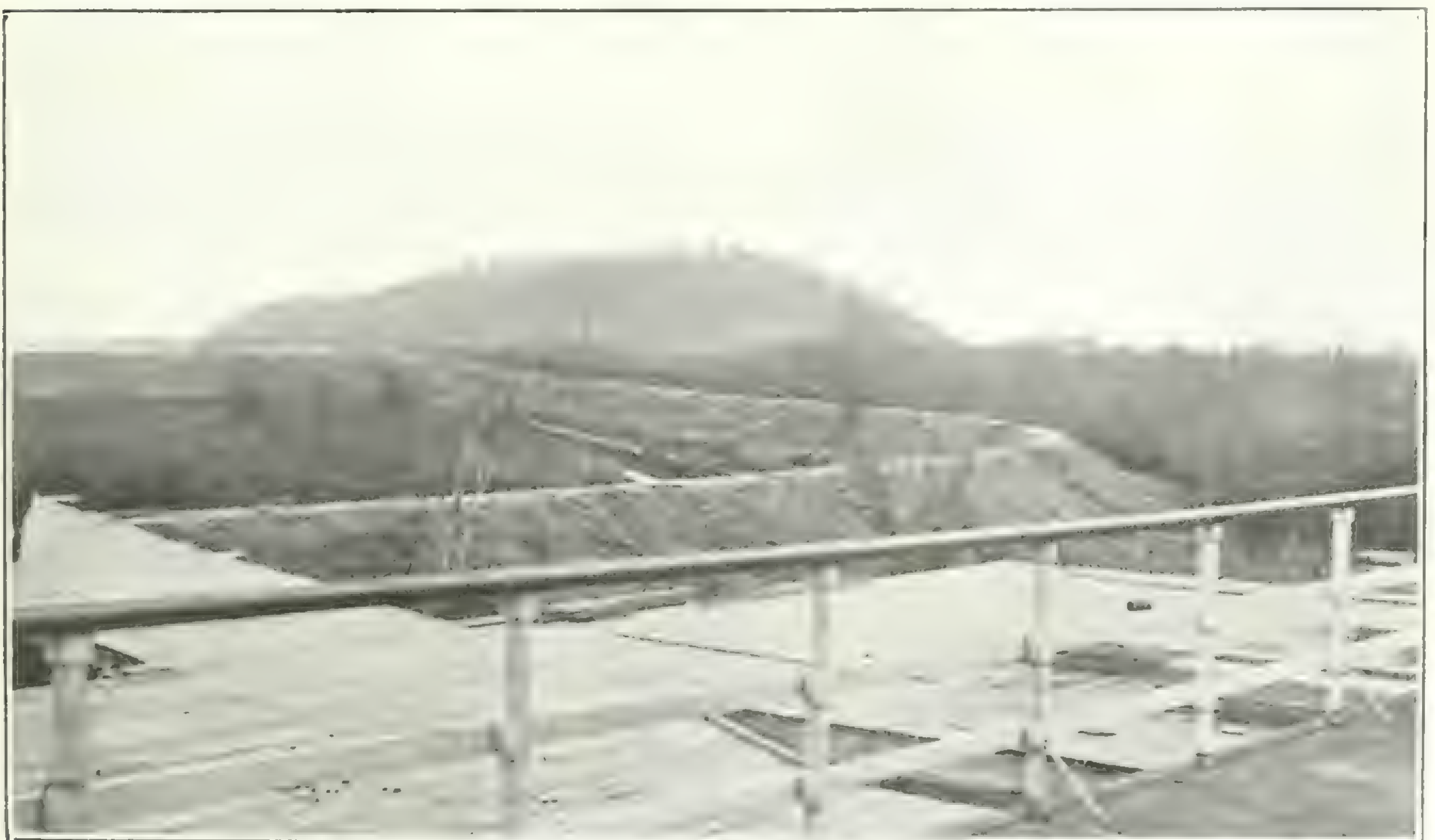
Reclamation-Pitt Meadows Dyke South of Sturgeon Slough.
